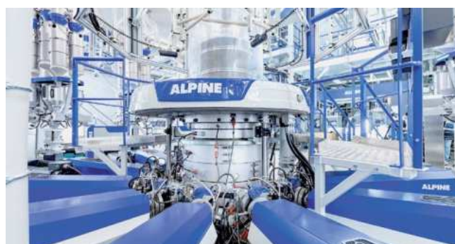
At the 9-layer blown film line in the modernised test centre in Augsburg, customers can work with Hosokawa Alpine to develop their ideal film formulation
